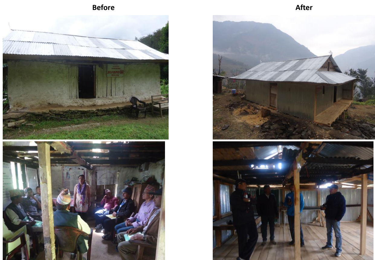
Figure 3.1: Before and after photos of infrastructure improvements at Khejenim SHP
